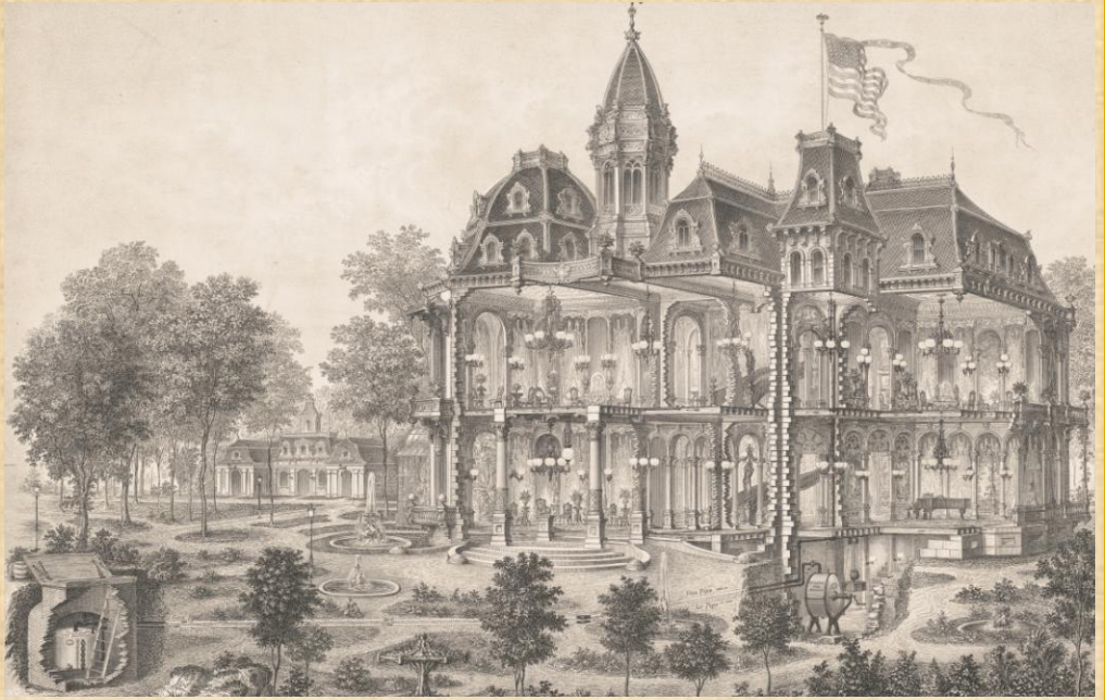
A depiction of an installation of the Springfield Gas Machine, the most widespread of such devices. Zoom in to note the underground vault containing the gas generator connected to an air pump in the mansion's basement.
